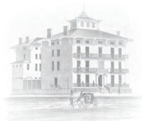
Scovill House in Waterbury
