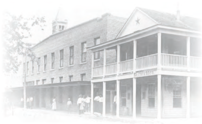
Post Office in Hallettsville
