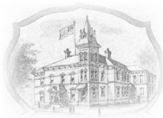
The High School in Enfield
